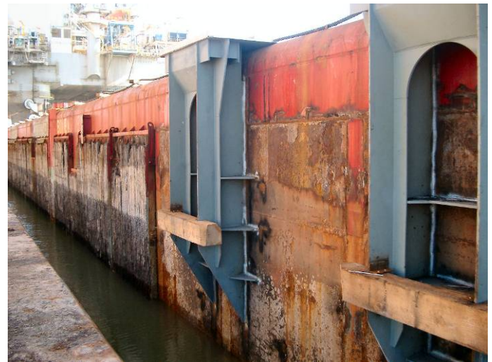
Figure 8. Support brackets welded to barge hull.
