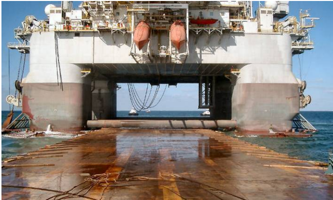
Figure 17. Barge pulled out from under rig braces.
