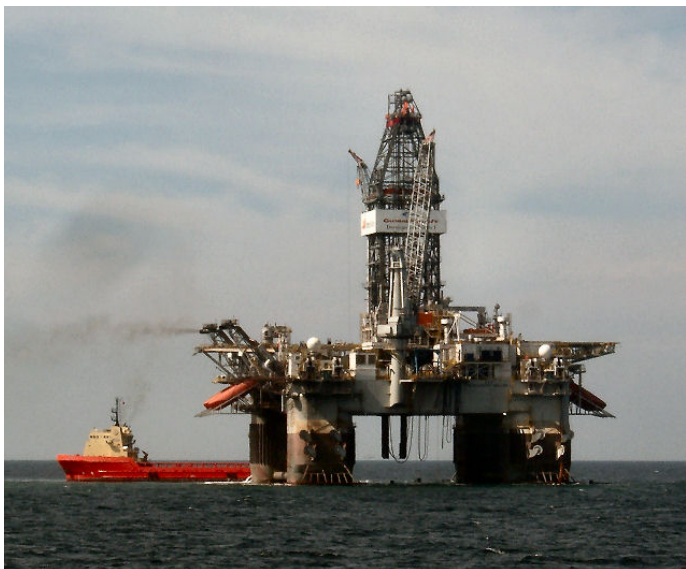
Figure 18. Rig taking on fuel and water from a supply vessel.
